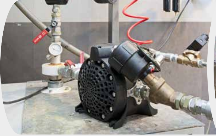
Cement additive dosing.
