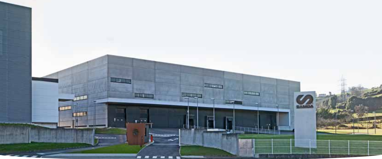
Headquarters Offices and Technical Centre in Gijón (Spain)
